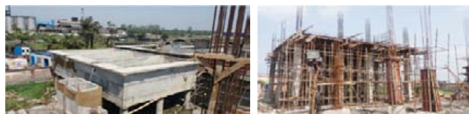
Sewerage System & STP works at Budge-Budge
