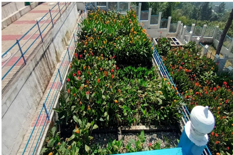
Figure: Actual view of the CWs at Dharamsala Near bus stand, Himachal Pradesh
