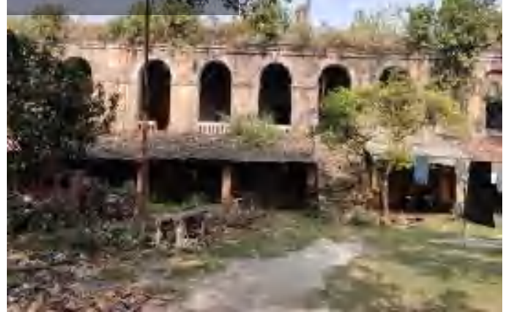
Old Police Station, Sabibganj
