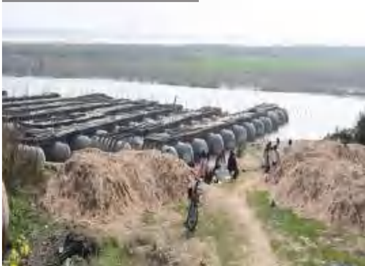
Incomplete Boat Bridge, connecting Ballia to Buxar
