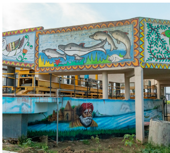
60 MLD Pahari STP in Bihar under Namami Gange Programme
