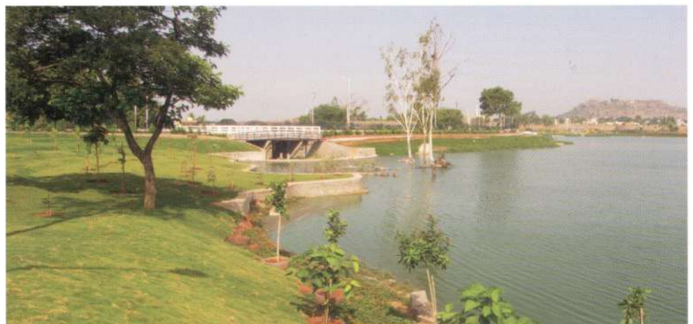
Restored surplus weir and bund - Langerhouz lake
