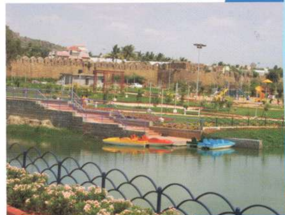
Langer Houz lake - after restoration
