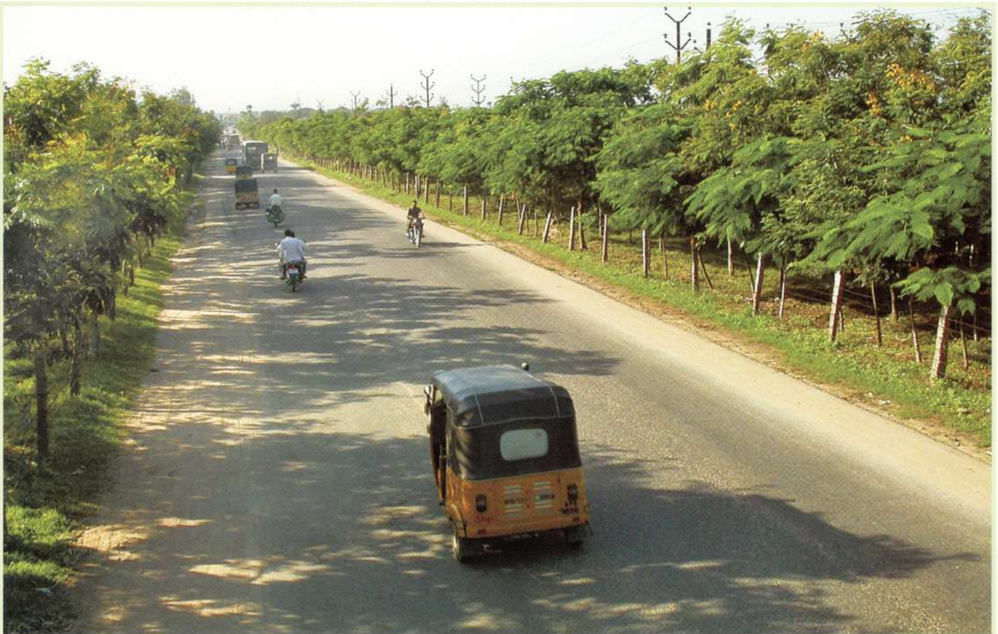
Green belts checking pollution - Narsapur road
