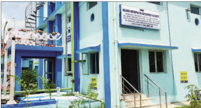
Budge Budge 9.3 MLD NJK (STP)
