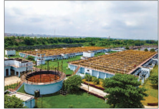
Rajapur, Prayagraj 90 MLD NJK (STP)
