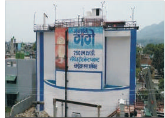
Chorpani 7.5MLD NJK (STP)
