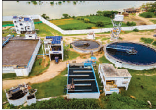
Kodra, Prayagraj 25 MLD NJK (STP)
