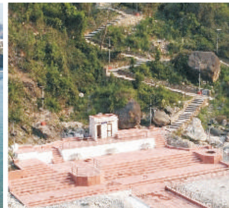
Renovated Ghat- 2, Rudraprayag
