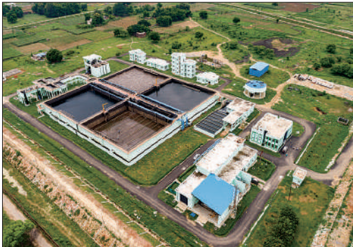
Ramanna, Varanasi 50 MLD NJK (STP)
