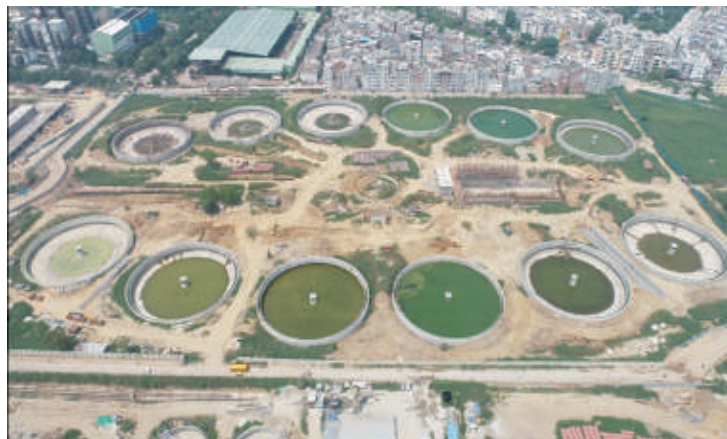
Okhla, Delhi 564 MLD NJK, STP
