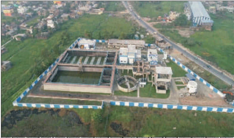
Barrackpore 24 MLD NJK (STP)
