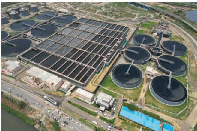
Coronation Pillar, Delhi 318MLD STP
