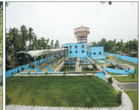
Bhatpara 41 MLD NJK (STP)
