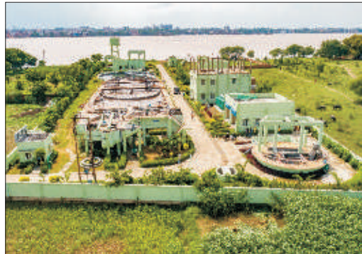
Ramnagar, Varanasi 10 MLD NJK (STP)
