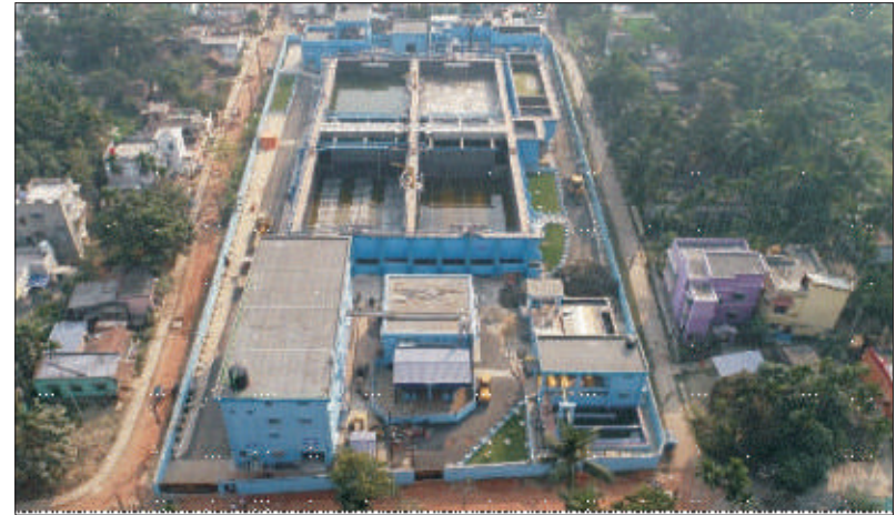
Hrishihar 16 MLD NJK (STP)
