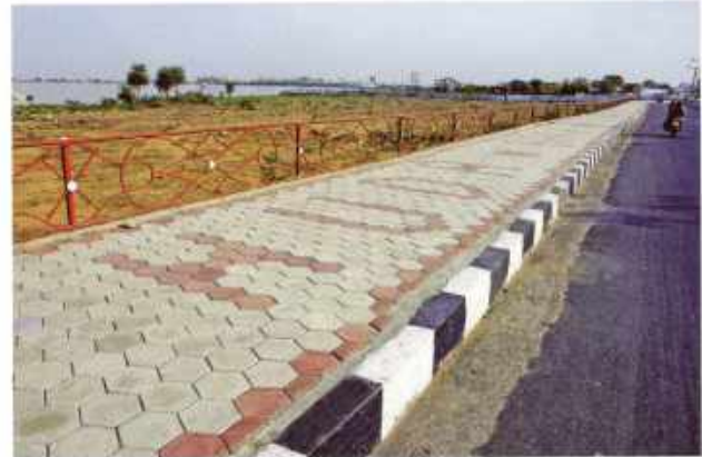
Pavement with Interlocking blocks on Necklace Road.
