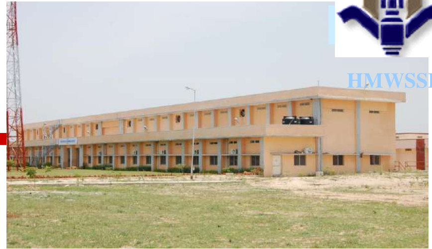
Pump House - Godakondla
