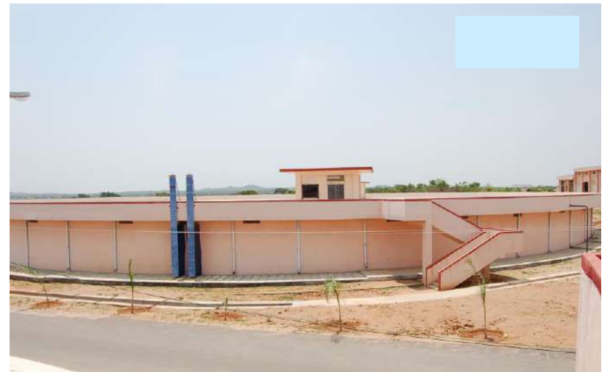
Over View of MBR - Gungal
